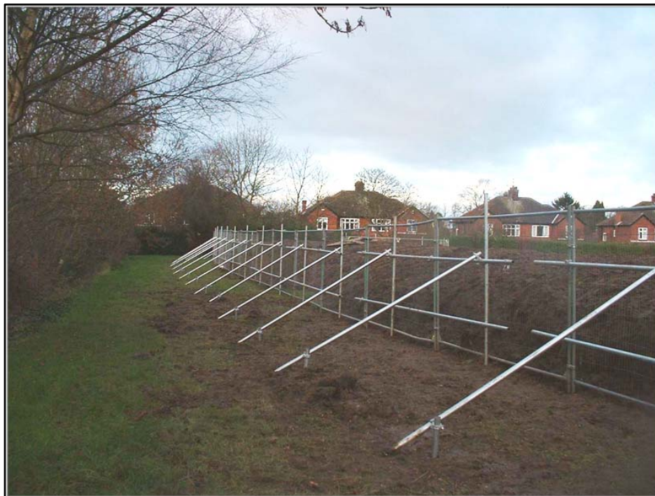
Figure 2- Actual barrier erected on site
